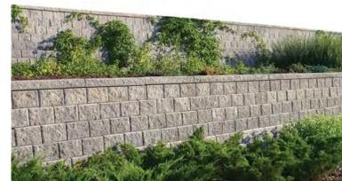
ORCO BLOCK CONCRETE MASONRY SPLIT FACE 8" MIN OR PER STRUCTURAL DESIGN WITH WALL CAP COLOR: NATURAL GRAY MEDIUM HEIGHT
