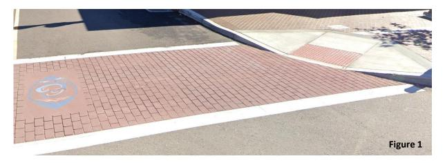
Similar decorative treatments on adjacent sidewalk areas are also observed at these locations, as illustrated by Figure 2 below. The decorative sidewalk areas appear to be actual bonded brickwork, as opposed to the Bomanite color stamped concrete utilized for the crosswalks.
