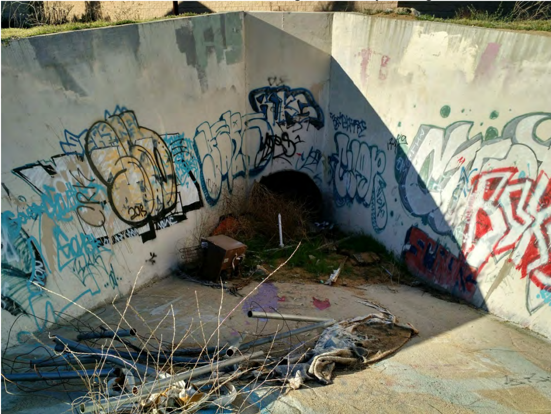
Inlet Headwall with Debris Blockage near Canyon Ridge Drive
