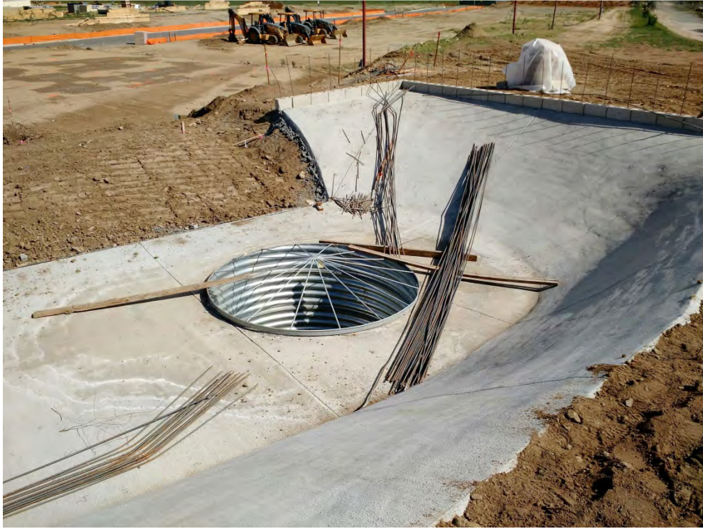
Image 18 Storm Drain Inlet in a Detention Basin off Hermosa Drive
