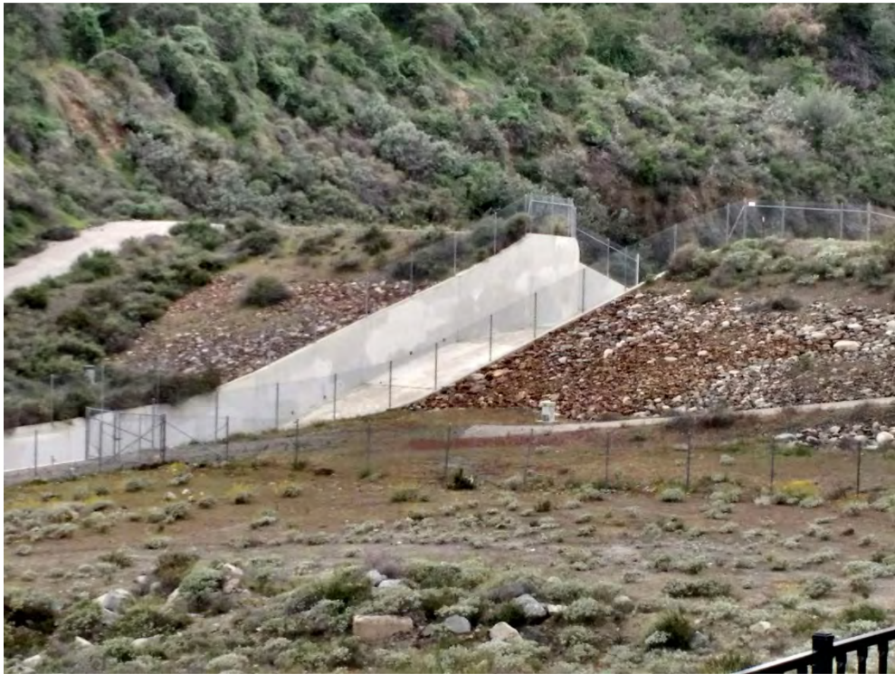
Image 23 Large Overflow Weir atop Culvert near Canyon Hill Community Park
