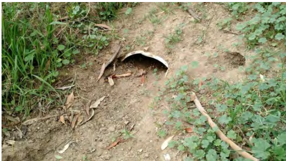
Storm drain outlets blocked with dirt on Pierce and Collier Avenue
