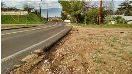
Dirt shoulder erosion adjacent to pavement on Franklin Street
