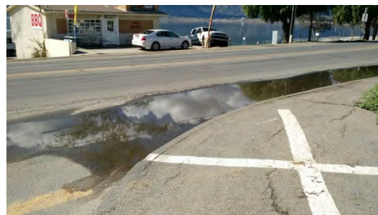
Roadway flooding on Lakeshore Drive at Match Street
