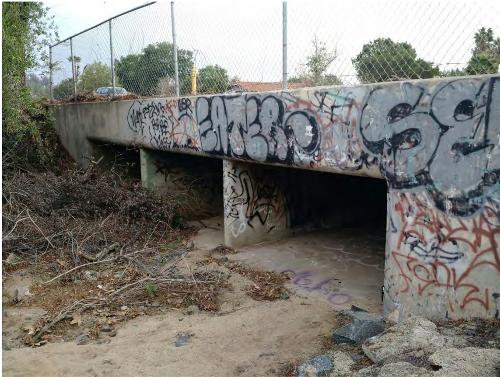
Image 20 Box Culvert underneath Collier Avenue with Sediment and Debris
