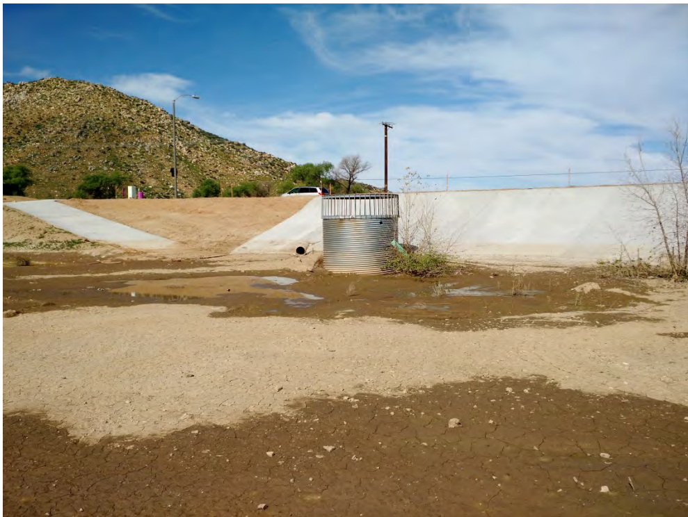
Image 18 Storm Drain Inlet in a Detention Basin off Hermosa Drive
