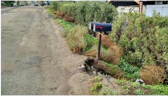
Street flow on Ellis Street drains down slope into property at Lower elevation
