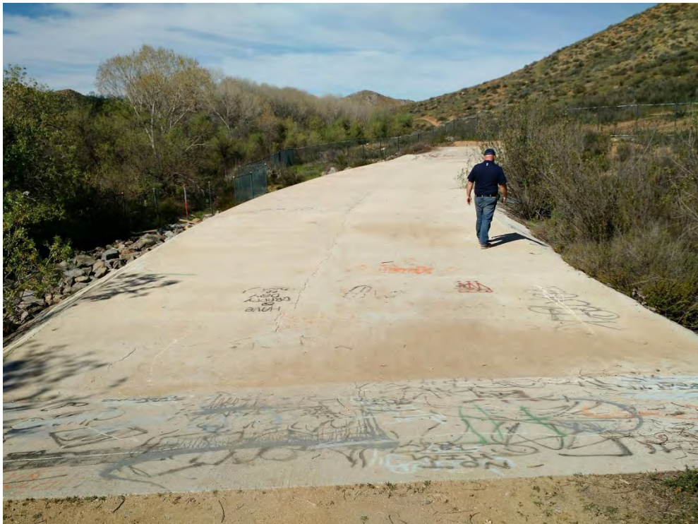
Image 23 Large Overflow Weir atop Culvert near Canyon Hill Community Park
