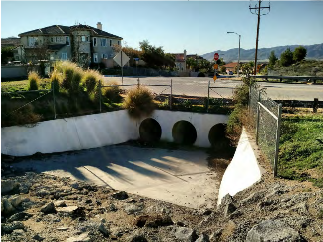
Image 19 3x54" Culvert underneath Canyon Estates Drive
