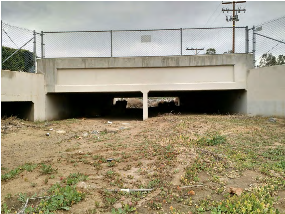
Image 20 Box Culvert underneath Collier Avenue with Sediment and Debris
